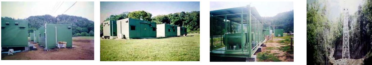
FIXED STATION RADAR SURVEILLANCE & TOWER
