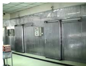
COLD STORAGE ROOM
